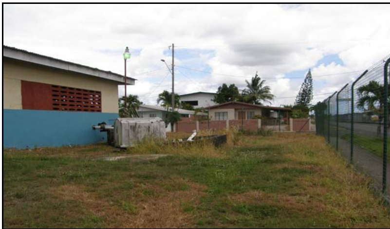
Photograph 3.7: Malabar Lift Station
