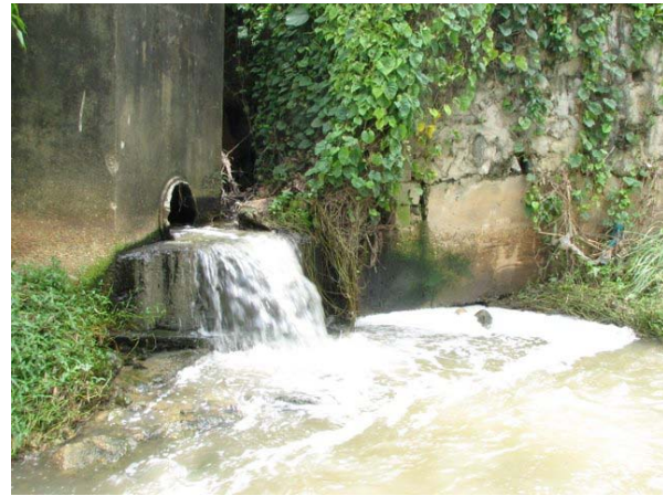
(j)WTP2 Arima WWTP (effluent into Mausica River)
