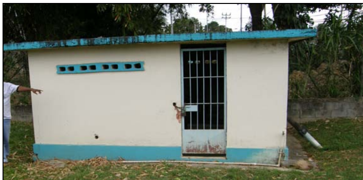
Photograph 3.5: Darceuil Lift Station
